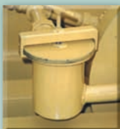
Easy Access Basket Strainer Reduces Tip Clogging
